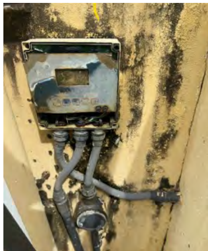
Figure 15: Parshall Flume Level Transmitter
