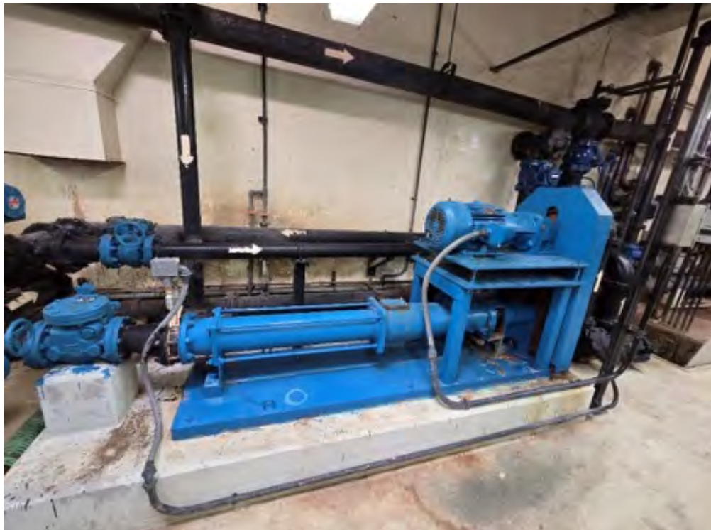
Figure 46: Centrifuge Feed Pump 2
