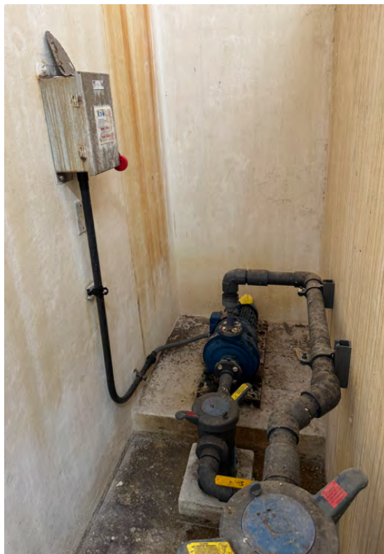
Figure 54: Chemical Transfer Pump (CTP)
