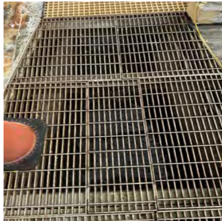
Figure 14: Parshall Flume on Diversion Channel
