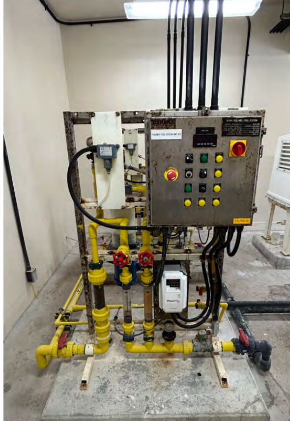
Figure 59: Polymer Feed System #2 (IPS-2)
