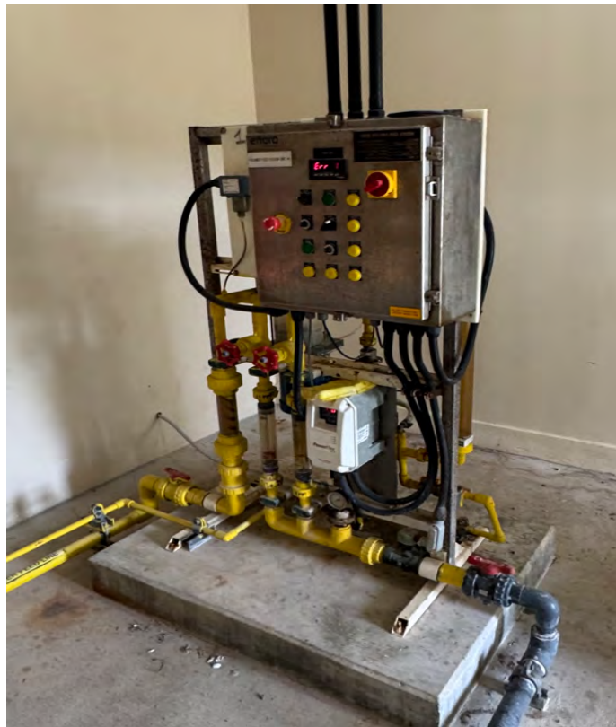
Figure 58: Polymer Feed System #1 (IPS-1)
