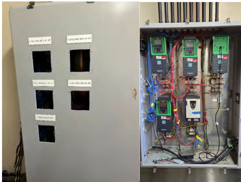
Figure 11: VFD Cabinet
