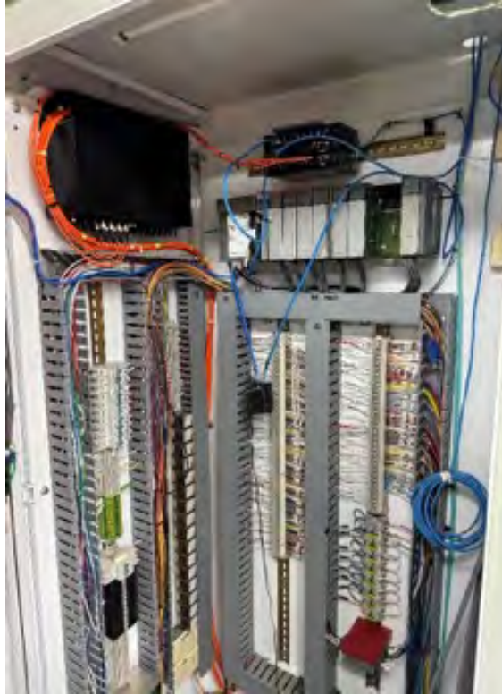
Figure 61: PLC-MST Interior
