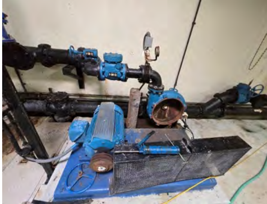
Figure 43: Dewatering Pump 1
