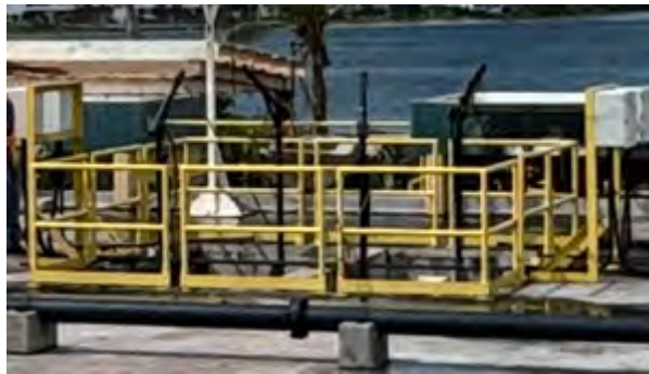
Figure 16: Flocculation mixers
