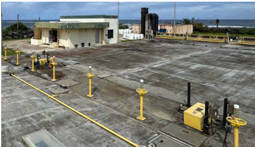
Figure 23: Sludge Collectors for Clarifiers 1 and 2
