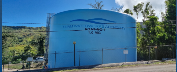
Picture of Agat No. 1 tank after the 1 MG steel water tank was fully repaired and coated. The Agat No. 1 Water Tank was completed and put into service in November 2023. This project ensures compliance with potable water standards, improves corrosion resistance, and extends the useful life of the water tank; enhancing system reliability and safeguarding public health.
