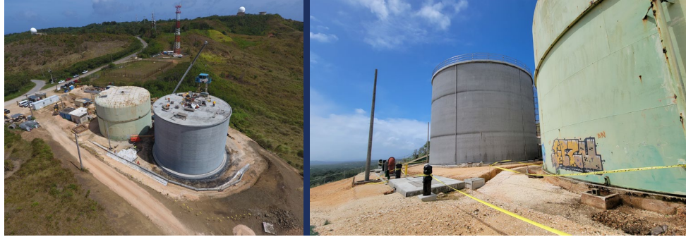
Attached photos are of the Santa Rosa #2 Concrete One Million Gallon (1 MG) Water Tank while under construction and the Santa Rosa #1 Steel Water Tank (1 MG) that was in service when these photos were taken. The Santa Rosa #2 Concrete Water Tank was completed and put into service October 2022, and the steel tank is offline and currently under repair.
