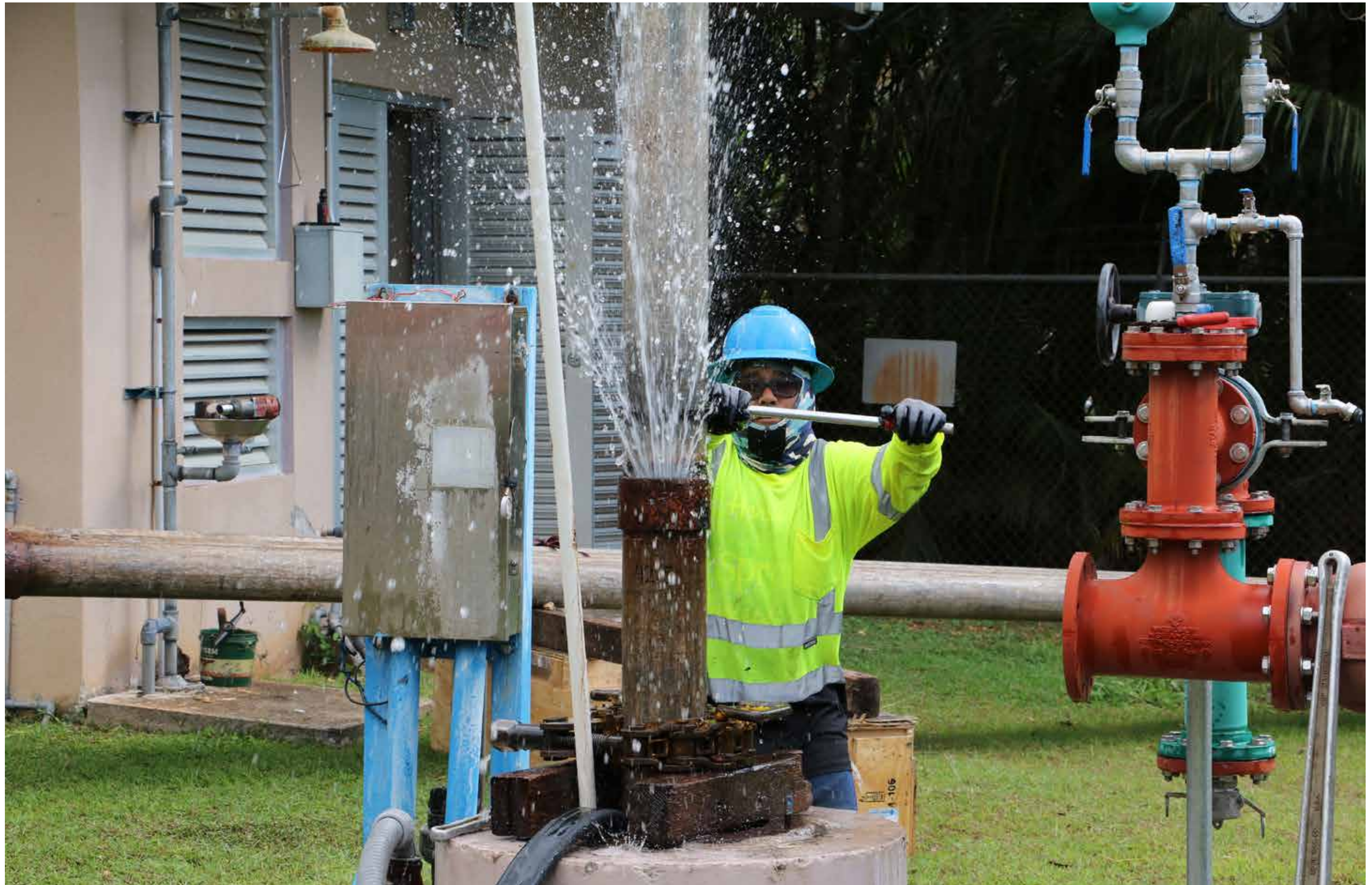
Utility Trades Helper Ryan Burgos of GWA's Deep Well Maintenance section disassembles a 500-ft deep pump discharge pipe column, one 25-ft pipe length at a time, releasing pristine groundwater in the process. The rest of the crew stand back to avoid the splash.
