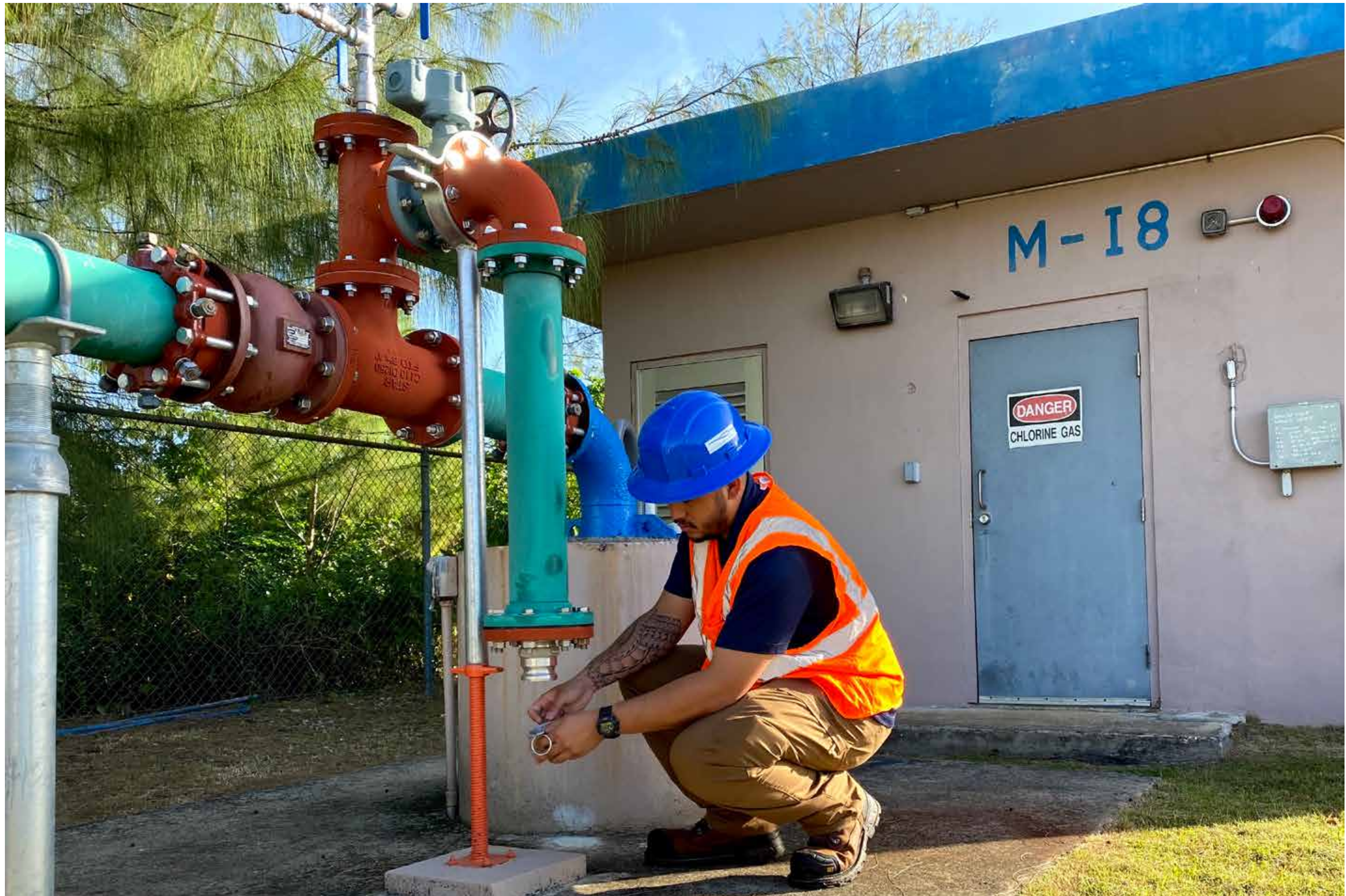
Water/Sewer Maintenance Worker I David Camaddu performs routine maintenance on one of GWA's more than 100 groundwater wells, which pump an average of 36-38 million gallons daily.
