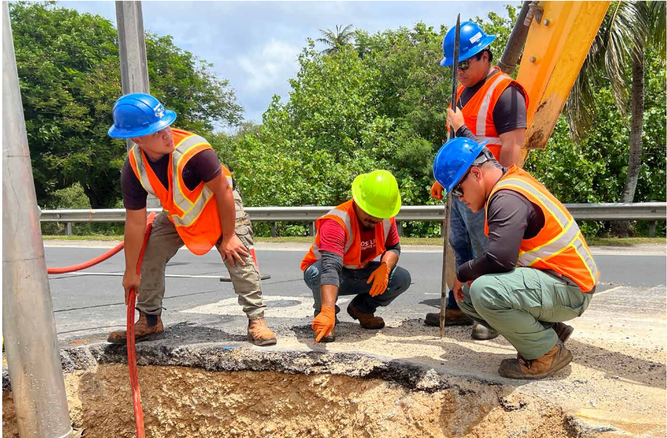
Lionel Chargualaf (green hat) of the Court Order unit work to hydro-excavate around delicate telecommunication utilities so Marcus Guerrero, Joseph Chargualaf and Keoni Duenas of GWA's Pressure Line Unit can make repairs to a leaking water distribution line without damage or disruption to communications services.
