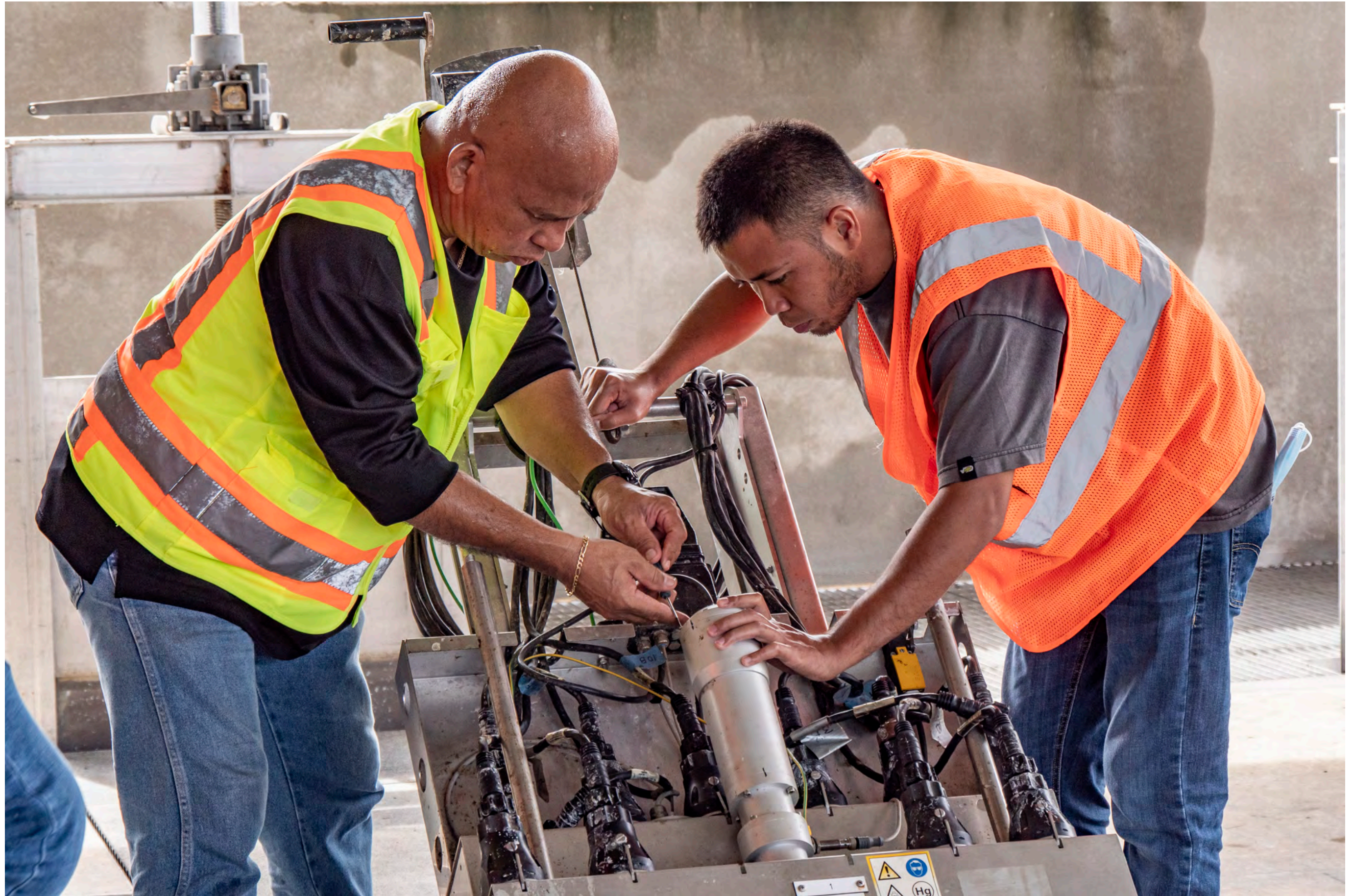
Benbenido Barcinas, Sewer Plant Supervisor, and Utility Trades Helper Kyle Taitingfong perform maintenance on UV disinfection equipment at the Agat-Santa Rita Wastewater treatment Plant.
