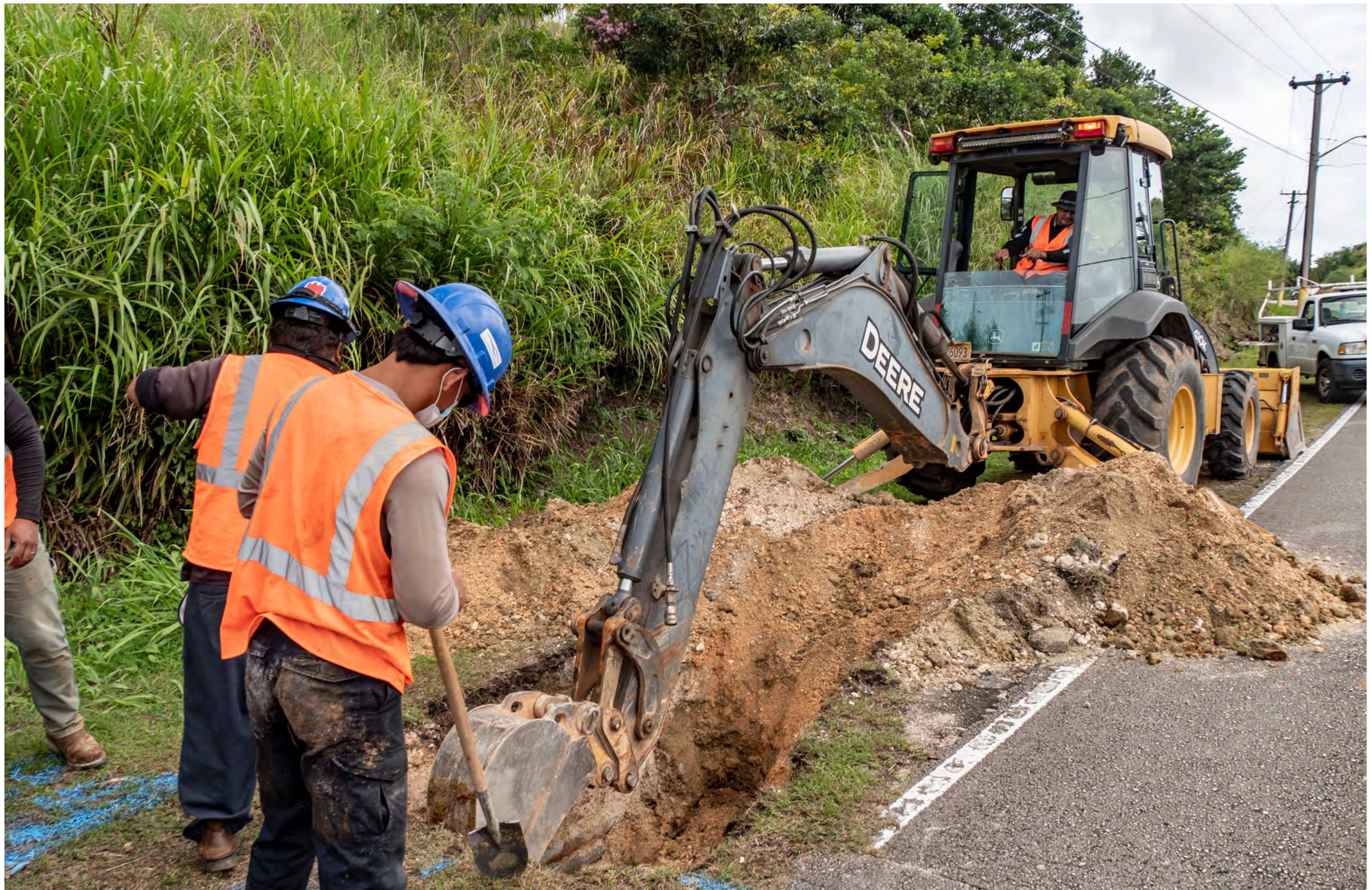
Water Distribution team members perform excavation to locate six-inch waterline and install a pressure reducing valve (PRV) vault.
