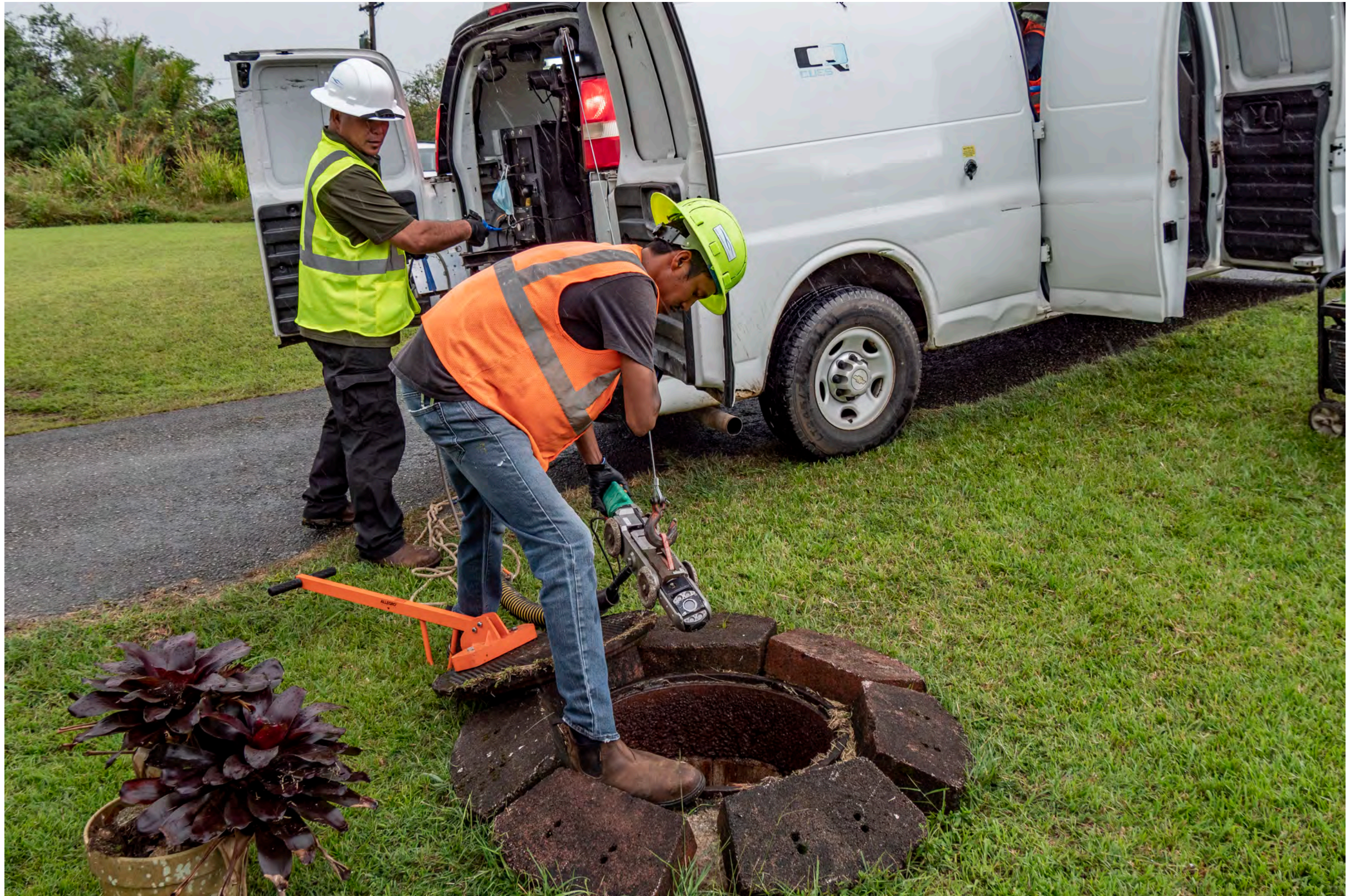
Water-Sewer Maintenance Worker Craig Paulino and Utility Trades Helper Edward Castro conduct CCTV inspections of sewer lines to detect and remove any potential blockage.
