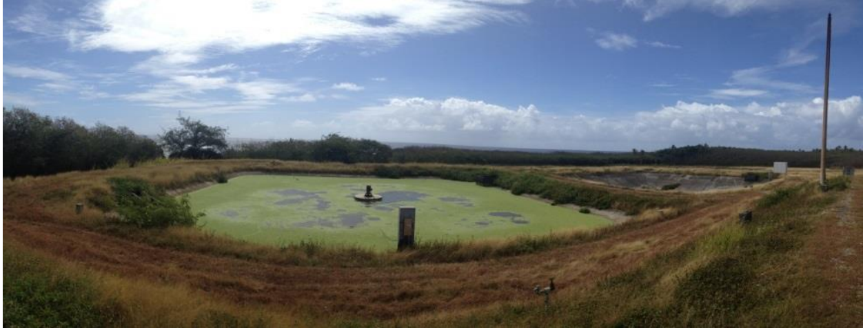
Figure 7-23. Inarajan WWTP Lagoons
