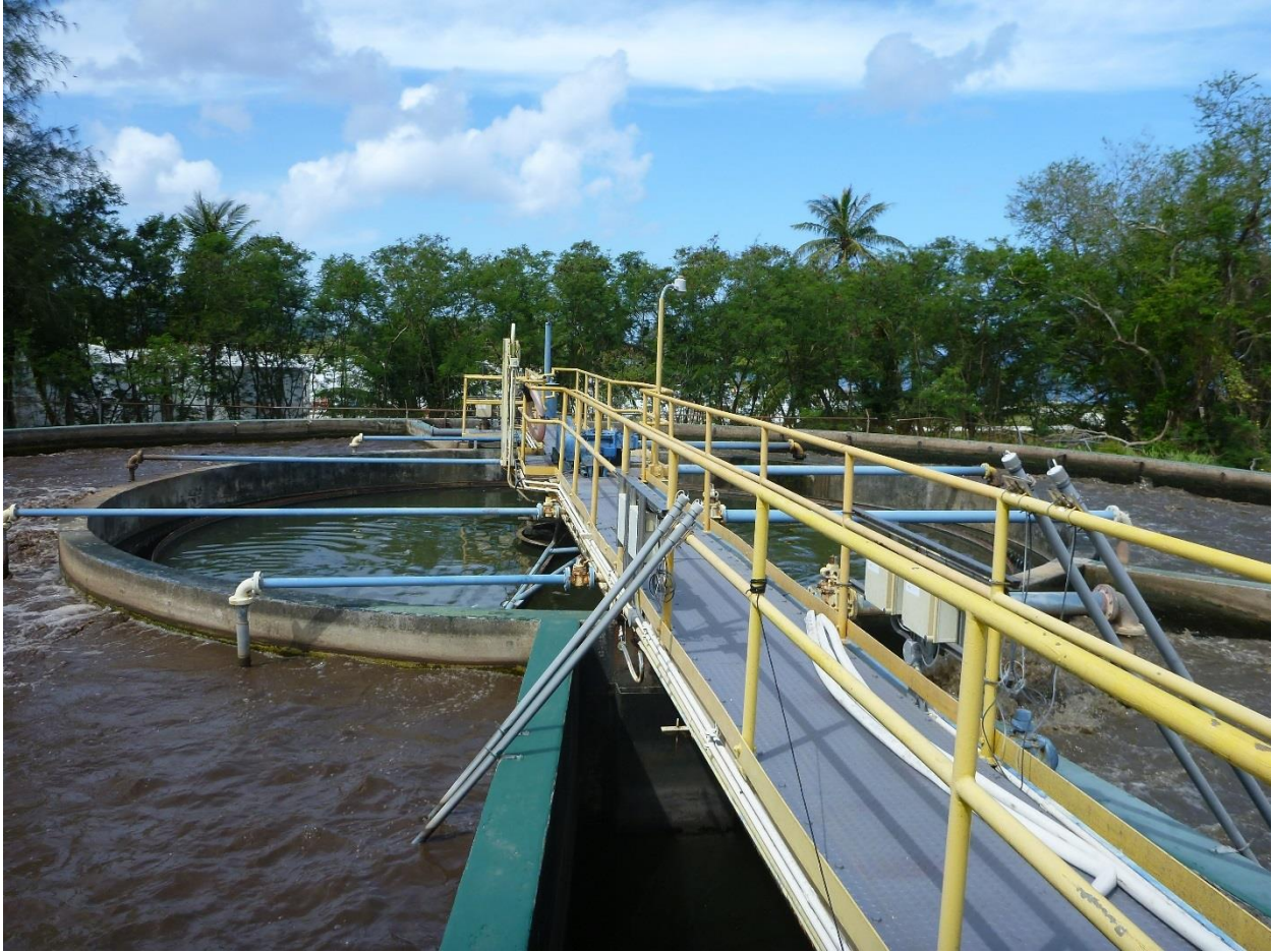
Figure 7-20. Existing Agat-Santa Rita WWTP (April 2010)
