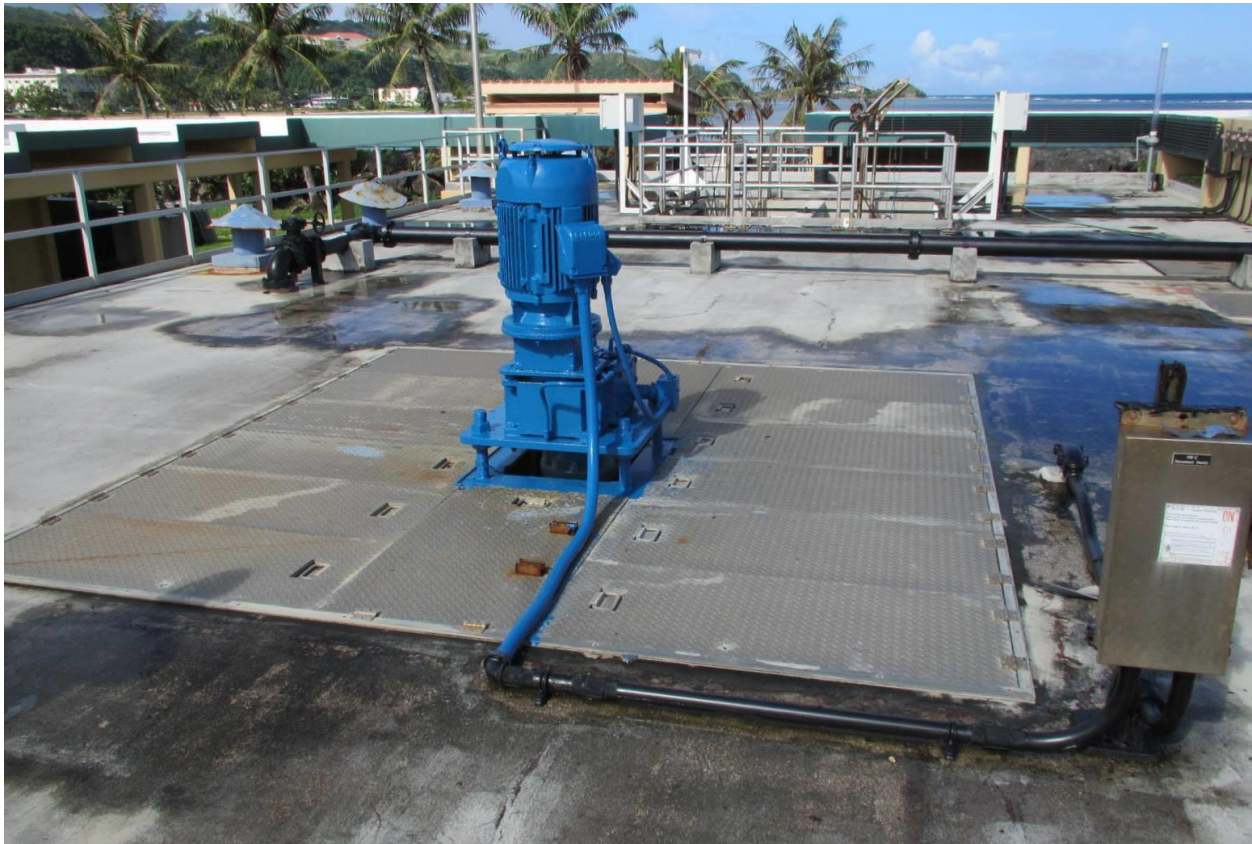
Figure 7-40. View at Hagåtña WWTP (October 2016)
