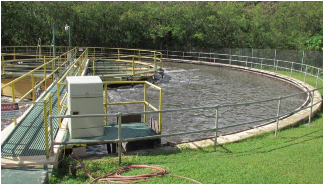
Figure 7-10. Baza Gardens WWTP (June 2013)
