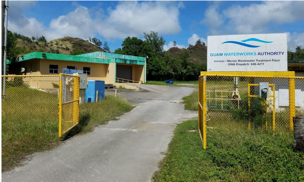
Figure 7-1. Umatac-Merizo WWTP (February 2017)
