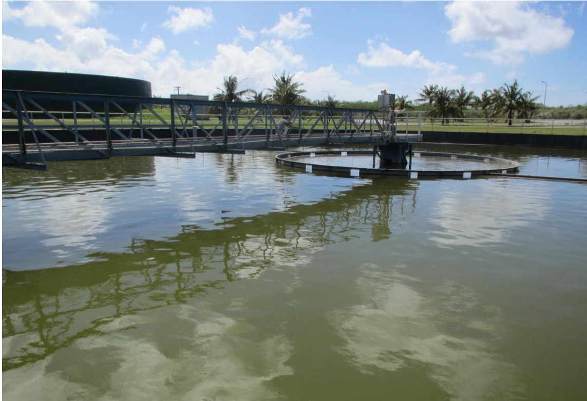
Figure 7-27. Northern District WWTP (February 2016)
