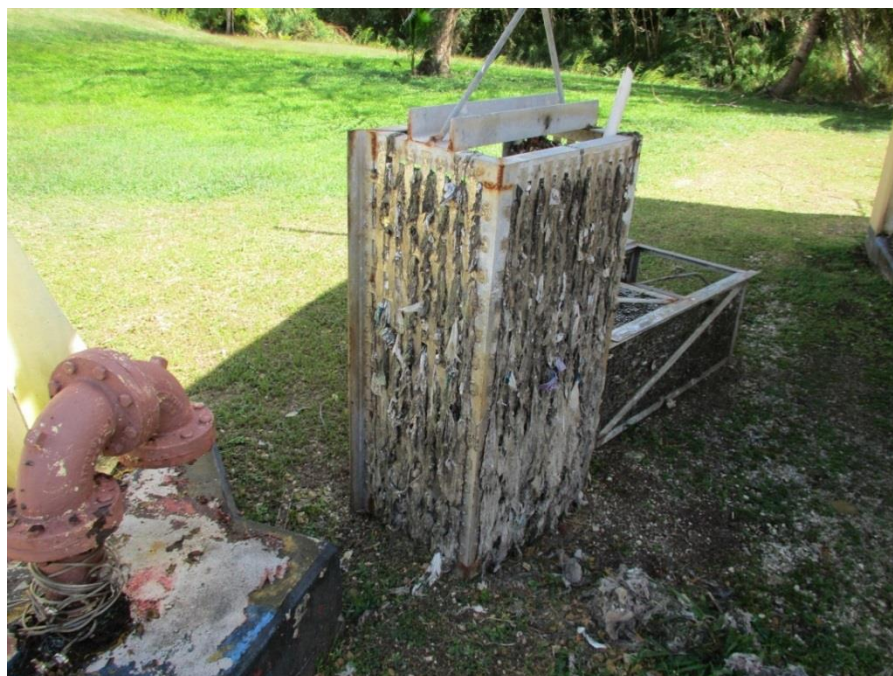
Figure 7-2. Umatac-Merizo WWTP Manual Basket Screen (January 2013)
