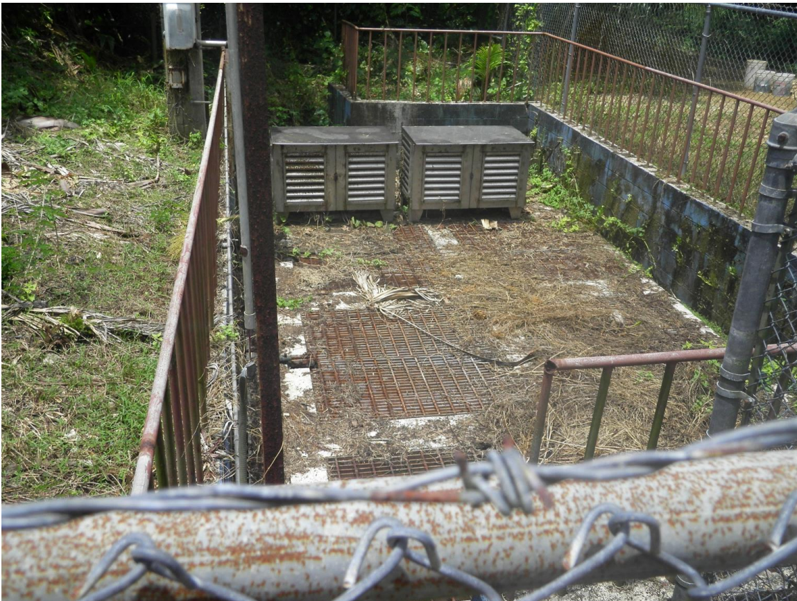
Figure 7-26. Pago Socio WWTP Blower Housing (2012)
