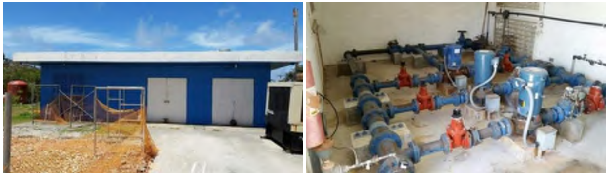
Figure B-6. Malojloj Elevated BPS Exterior and Interior
