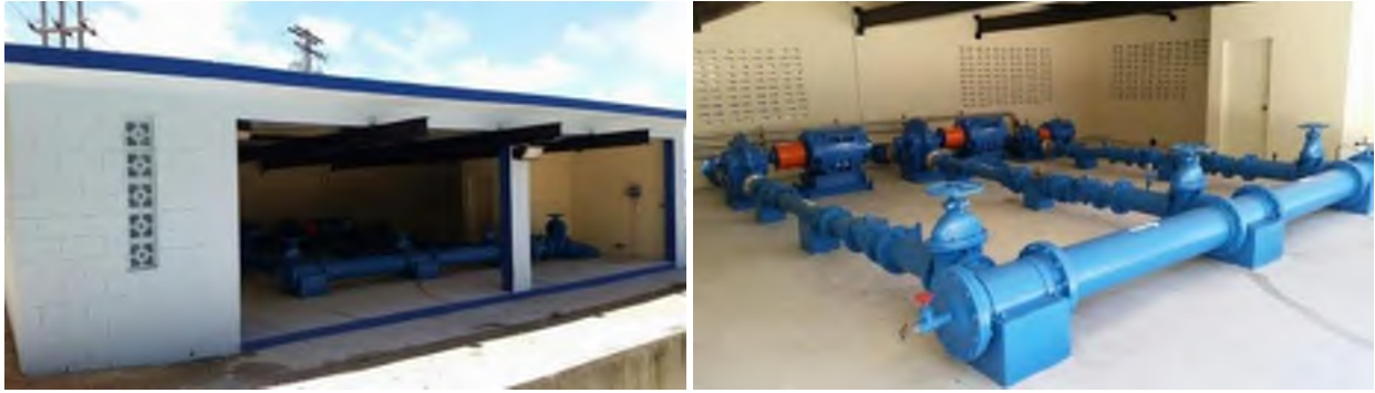
Figure B-10. Pago Bay BPS Exterior and Interior
