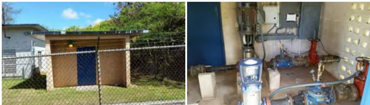
Figure B-15. Umatac 2 (WBP 2) BPS Exterior and Interior
