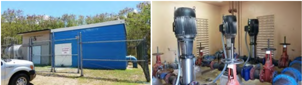
Figure B-2. Brigade BPS Exterior and Interior
