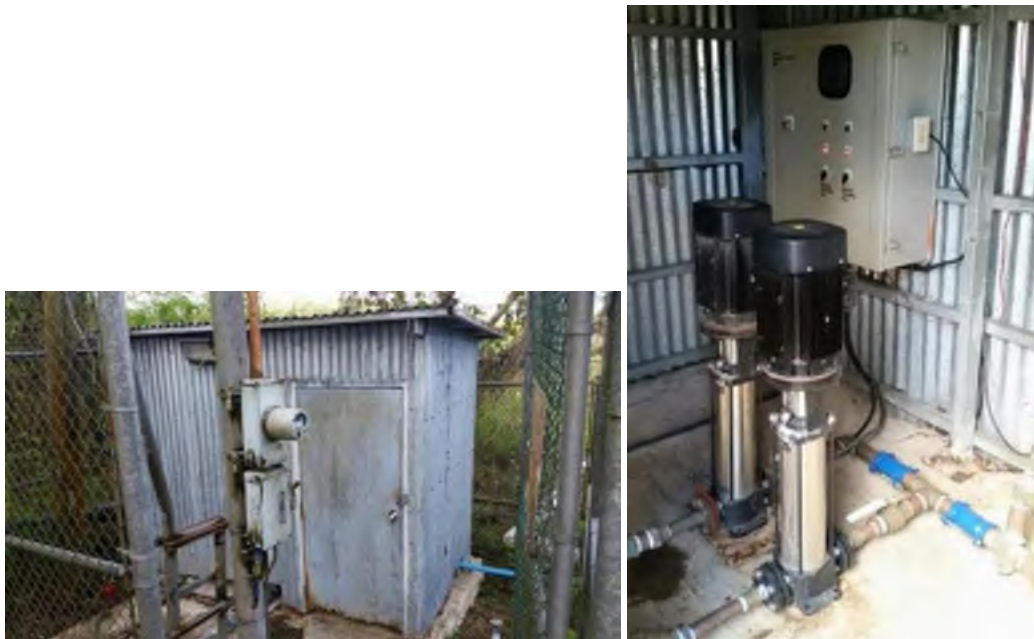
Figure B-9. Nimitz Hill BPS Exterior and Interior
