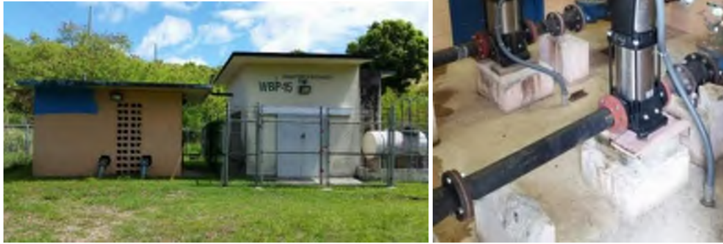
Figure B-13. Toguan BPS Exterior and Interior
