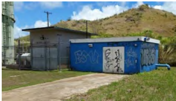
Figure B-12. Santa Rosa BPS Exterior
