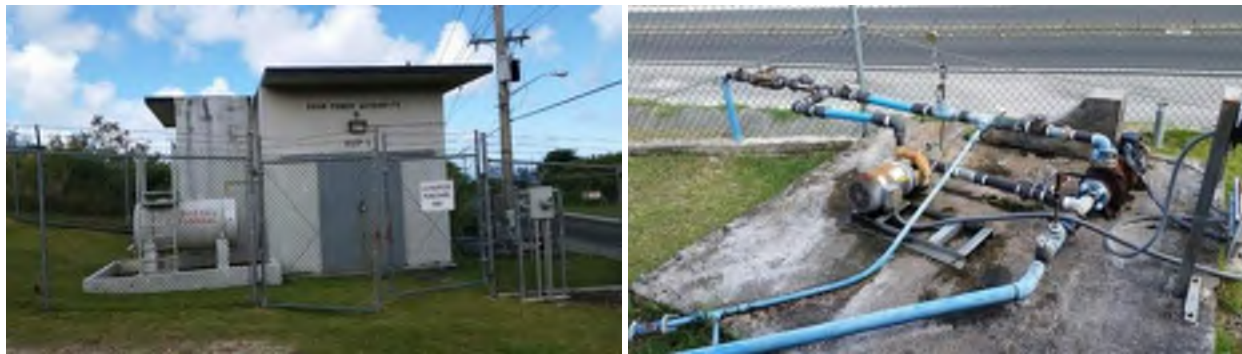
Figure B-14. Umatac 1 (WBP 1) BPS Exterior and Interior
