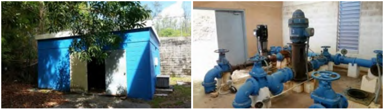
Figure B-11. Santa Ana BPS Exterior and Interior
