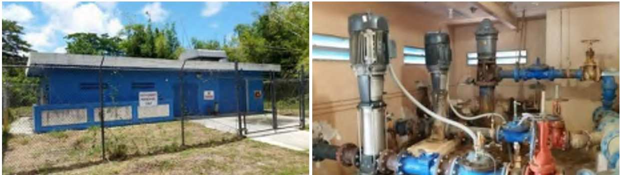
Figure B-1. Access BPS Exterior and Interior
