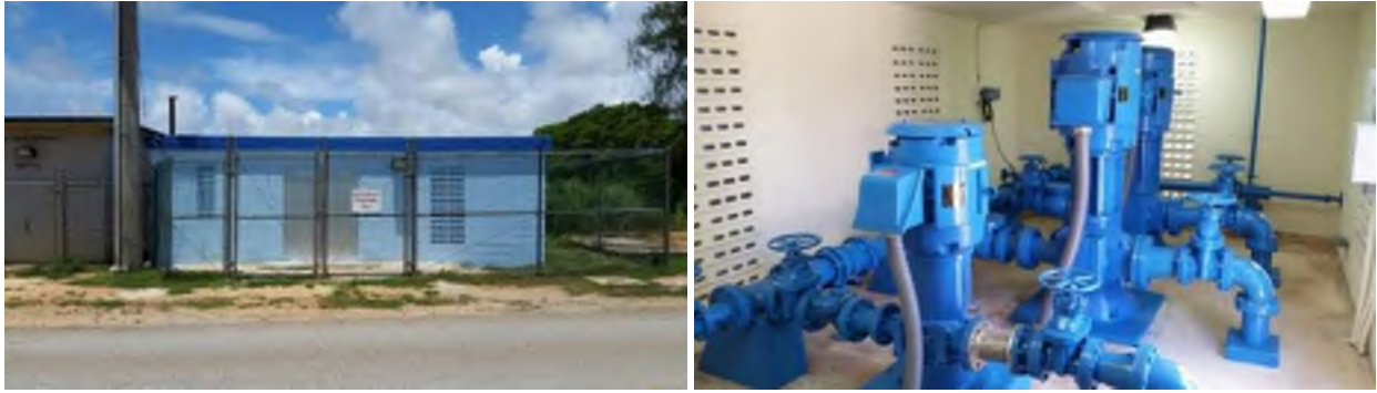
Figure B-16. Windward Hills BPS Exterior and Interior
