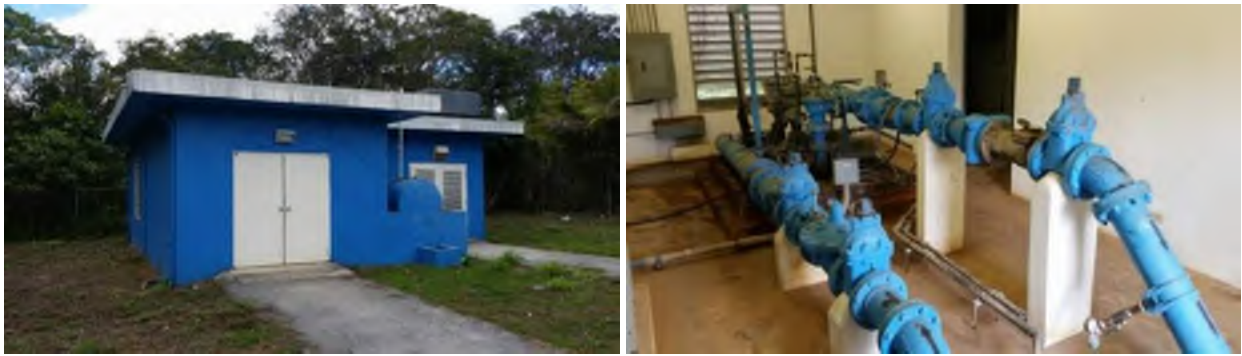
Figure B-8. Mataguac BPS Exterior and Interior
