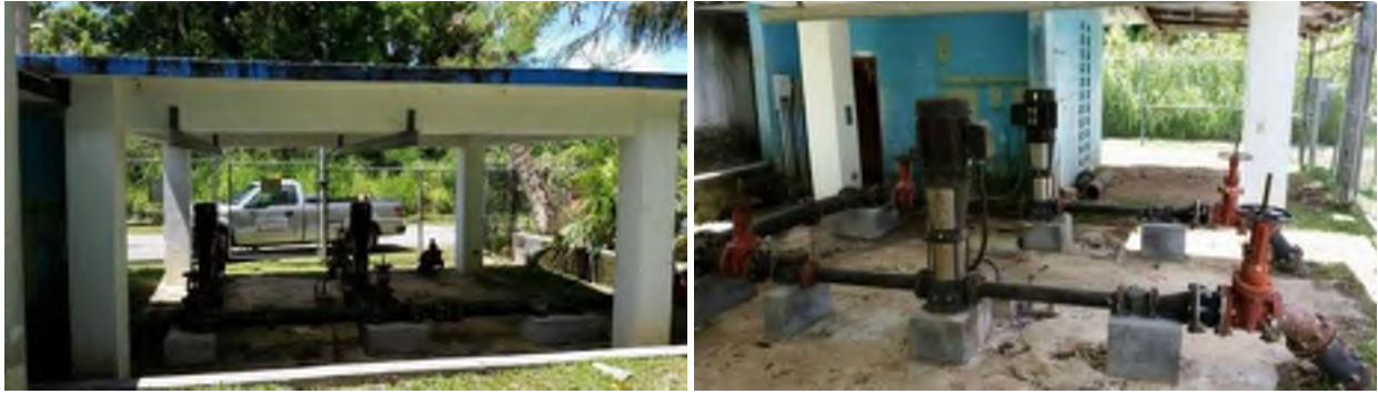
Figure B-4. Geus BPS Exterior and Interior
