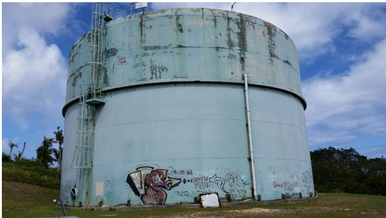
Existing tank in 2016
