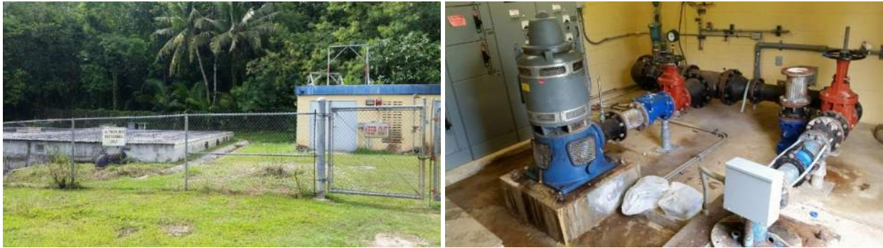
Figure 3-3. Santa Rita Spring Tank and Booster Pump Building (left) and Pumps (right)
