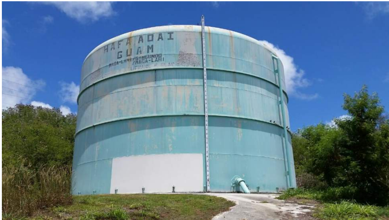
Existing tank in 2016
