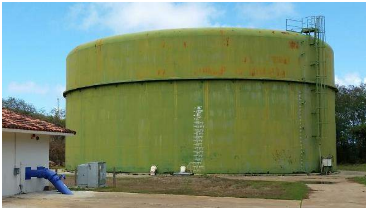
Existing tank in 2016
