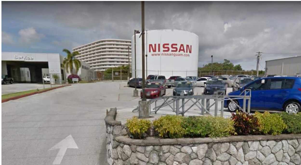
Existing, offline Nissan tank from Google Street View (2017)
