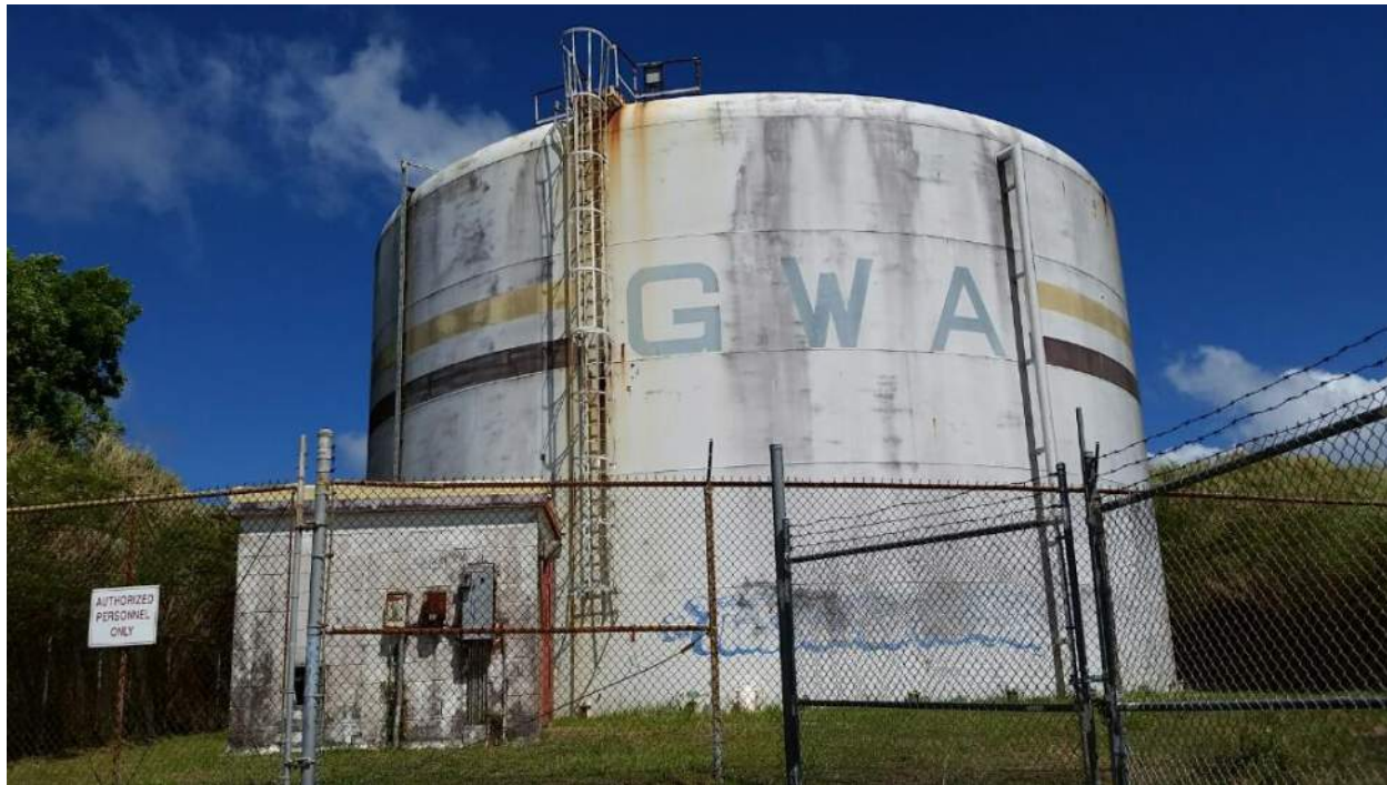
Existing tank in 2016
