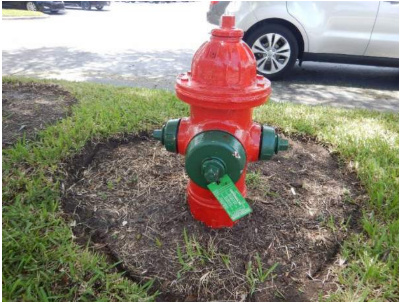
Figure 10-2. Fire Hydrant Color Coded by Fire Flow
