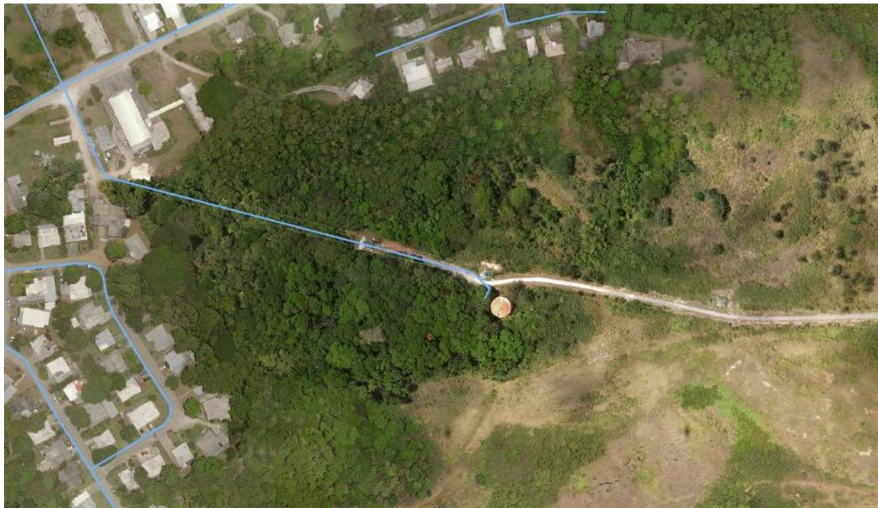
Existing tank from above
