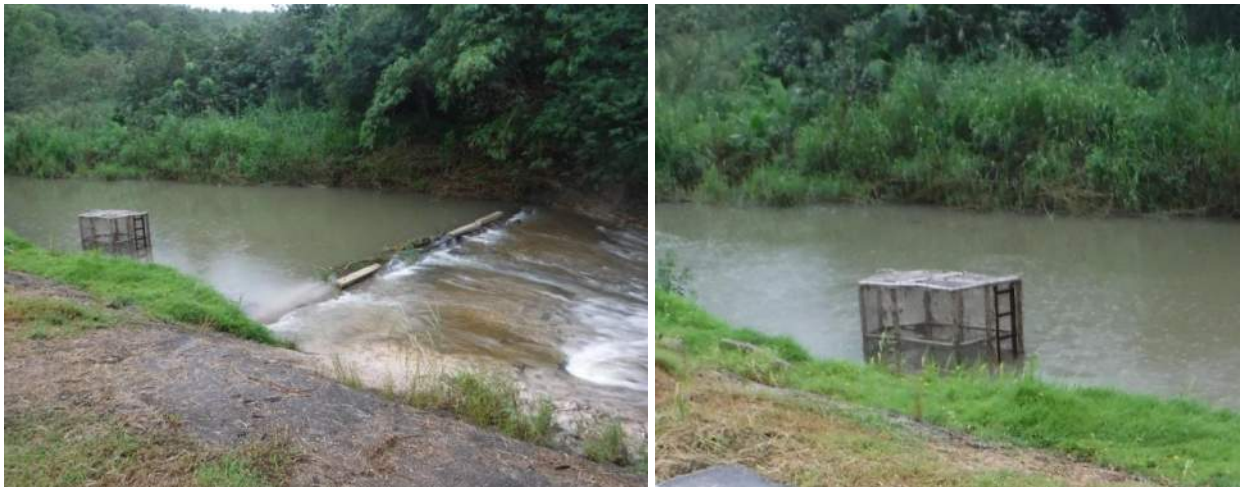
Figure 5-2. Dam with Stop Logs in Place (left) and Intake Screen (right)
