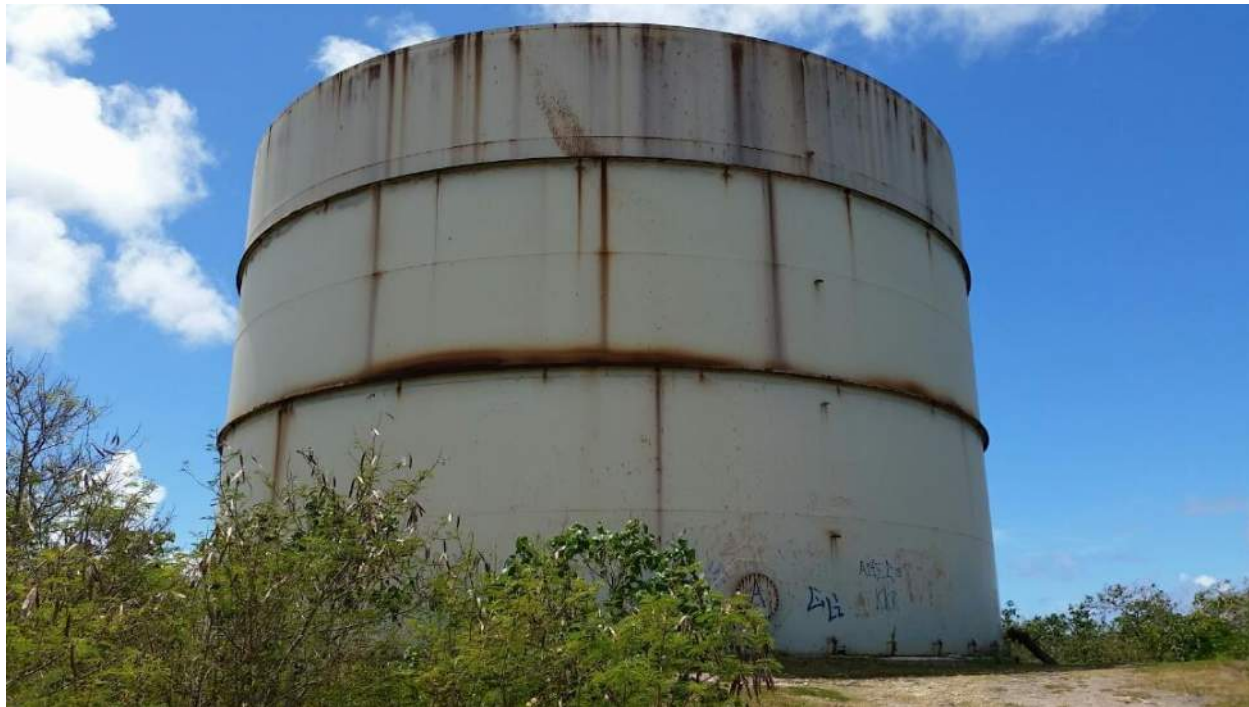
Existing tank in 2016
