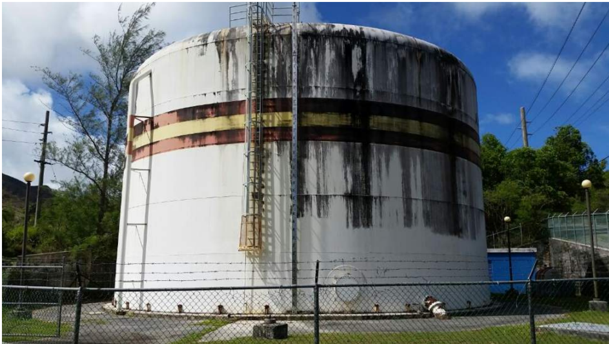
Existing tank in 2016
