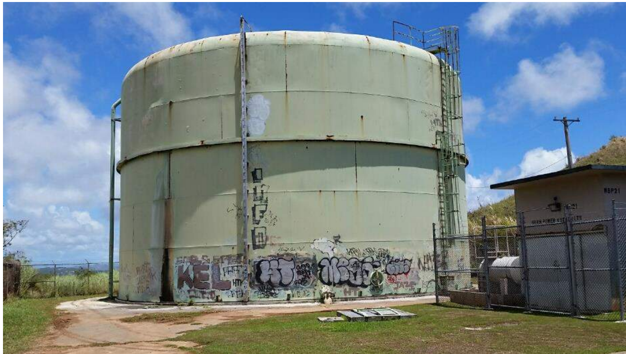
Existing tank in 2016
