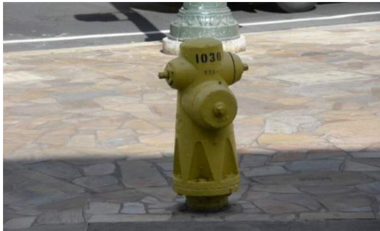
Figure 10-1. Fire Hydrant with Painted ID
