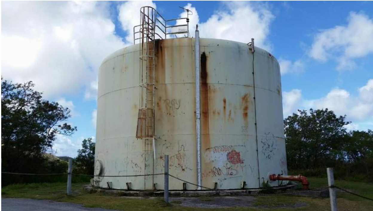
Existing tank in 2016
