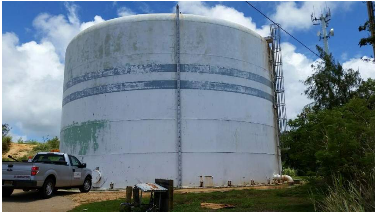
Existing tank in 2016
