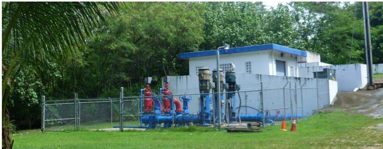
Figure 3-2. Raw Water Pump Station
