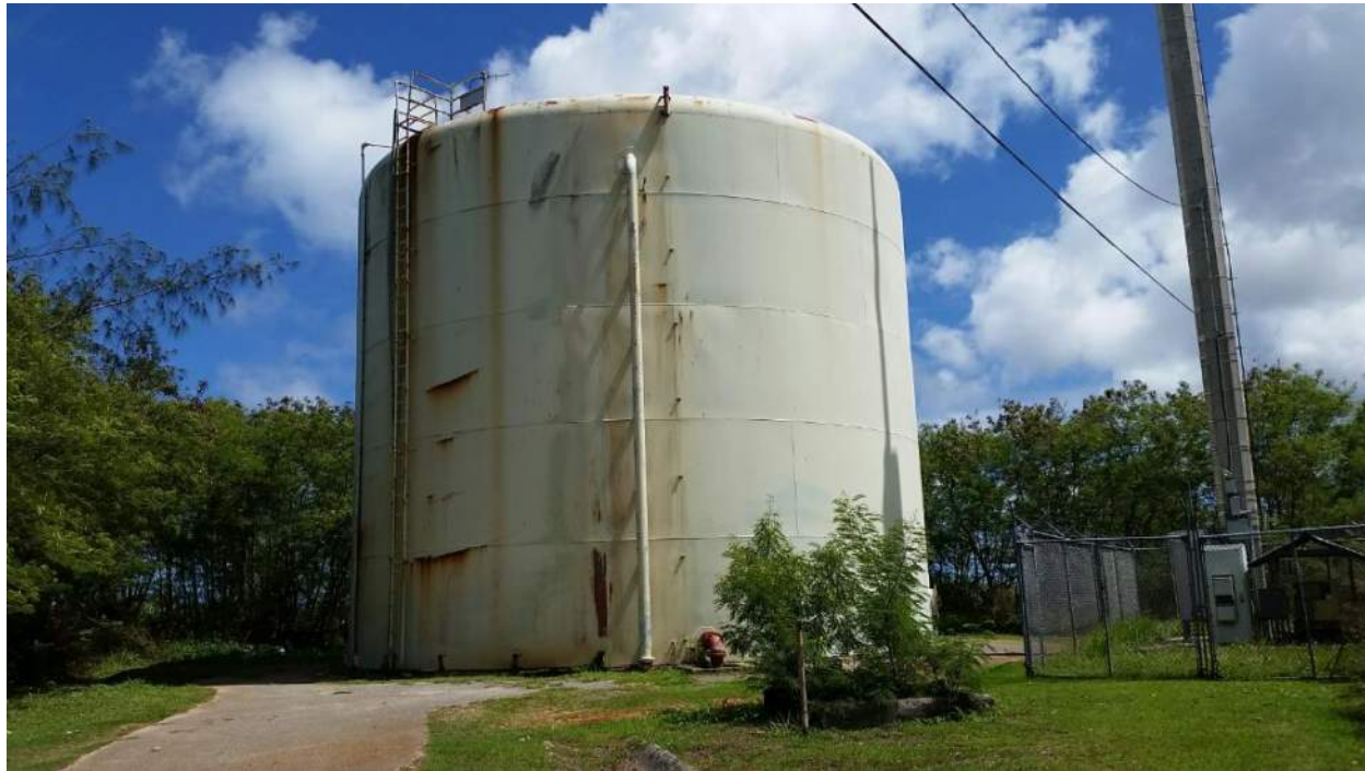
Existing tank in 2016
