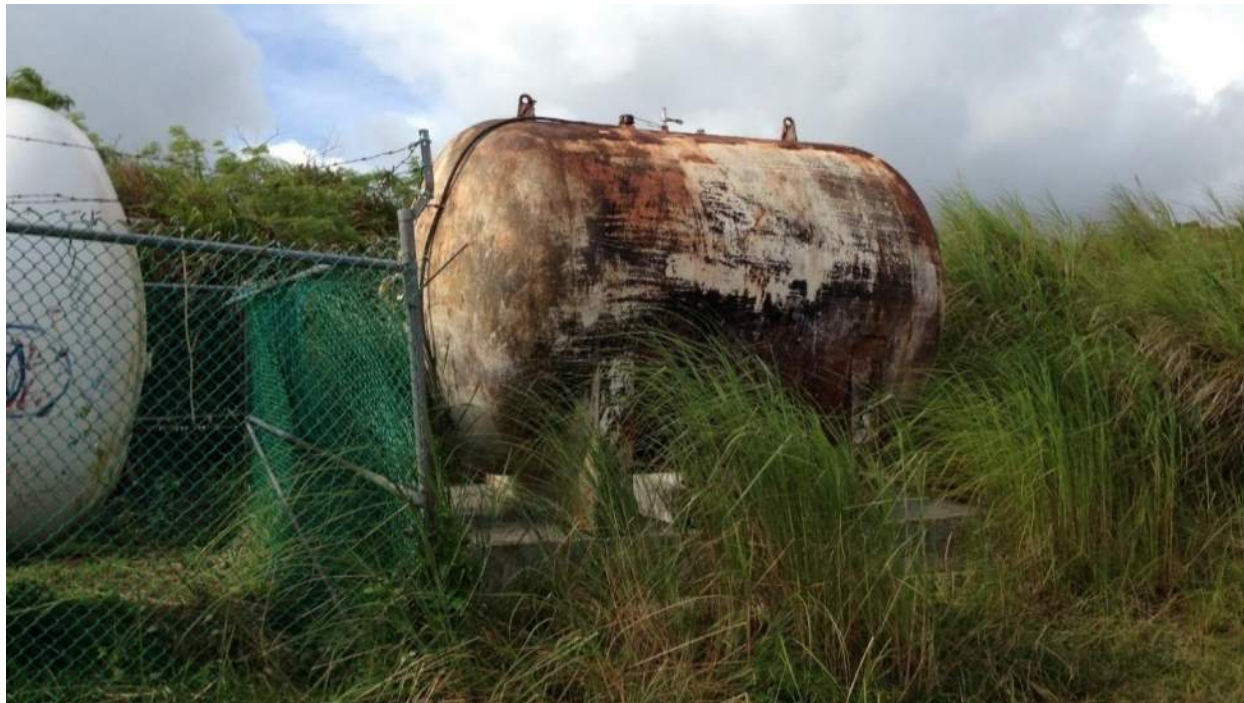
Offline existing old Lower tank next to Upper tank in 2013
