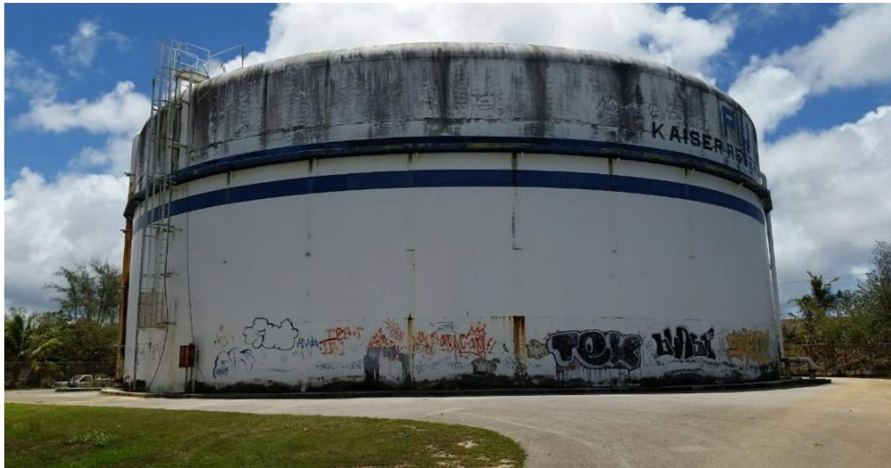
Existing tank in 2016
