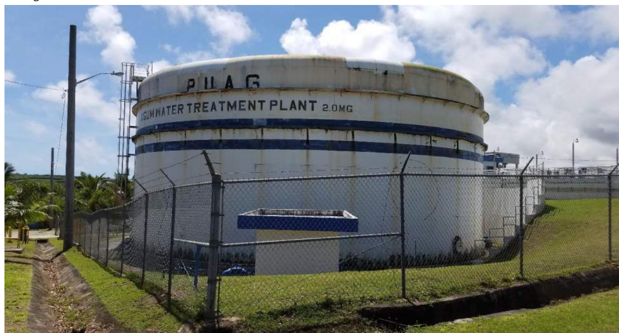
Existing tank in 2017
