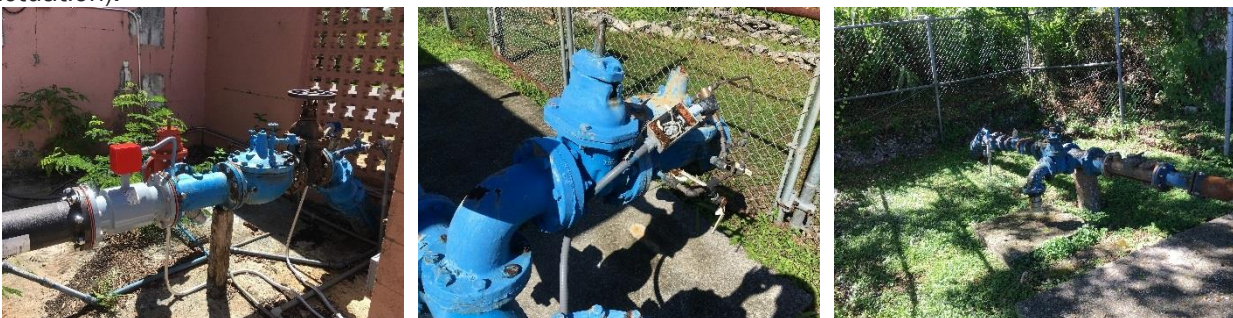
Figure 1-2. Well Discharge Piping at Wells A-1, A-18, and A-21
