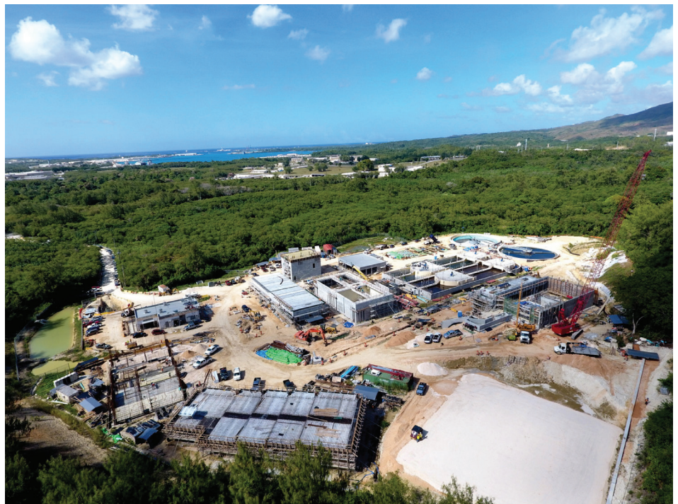
Agat-SR Wastewater Treatment Plant (Agat)
