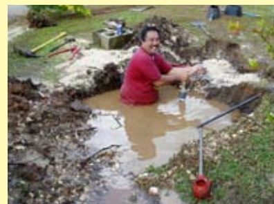
Ron San Nicholas, AMR Installation
