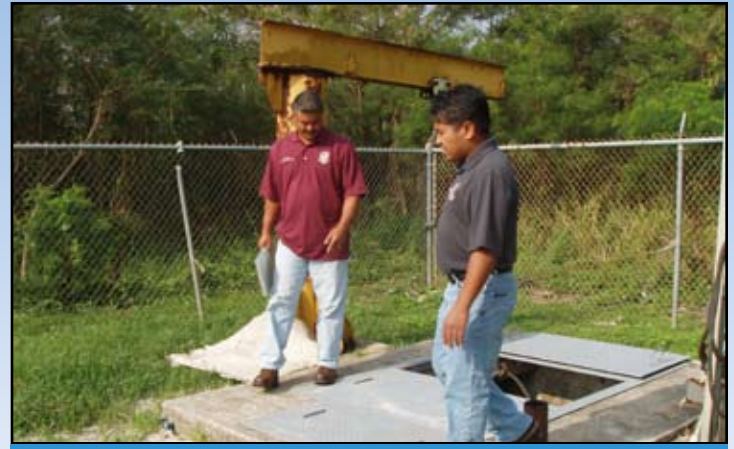
Vince Pangelinan and Jeffrey Borja at Dairy Road Sewage Pump station.
