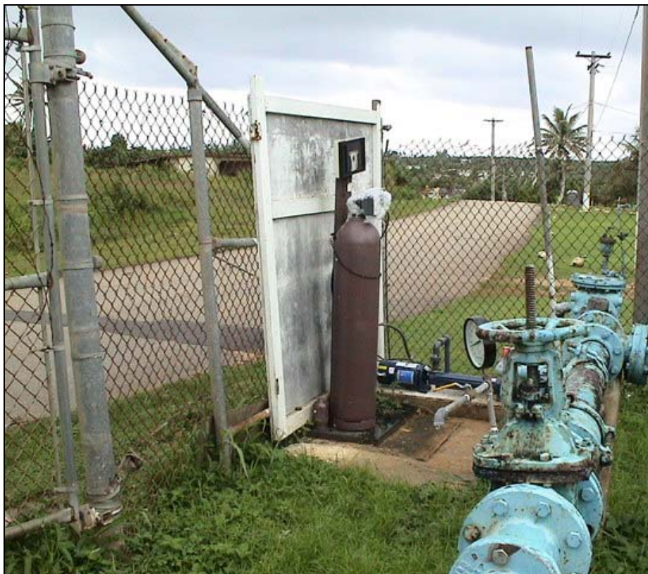
Figure 1-6 – Outdoor Chlorination System Installation
