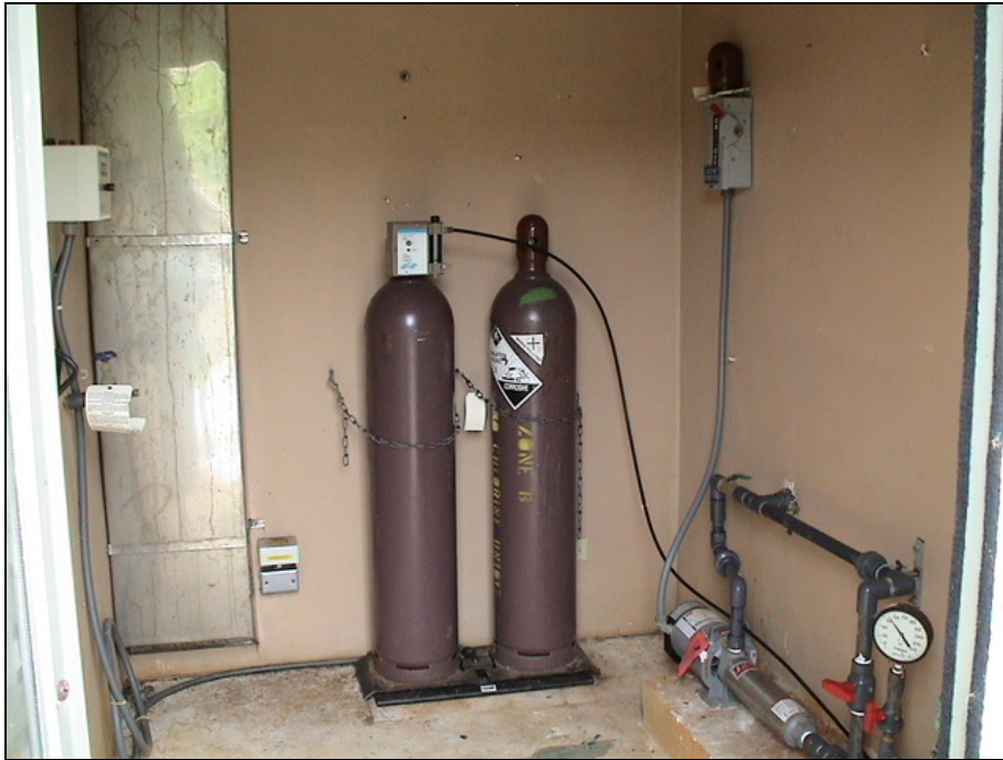
Figure 1-5 – Typical Well Indoor Chlorination System Installation
